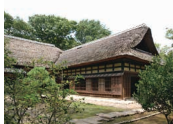
Omoya (Main building)
