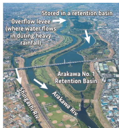
Arakawa No. 1 Retention Basin (Saitama and Toda cities, Saitama Prefecture)
